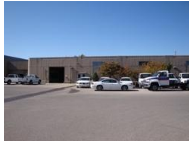
Light Equipment Shop
