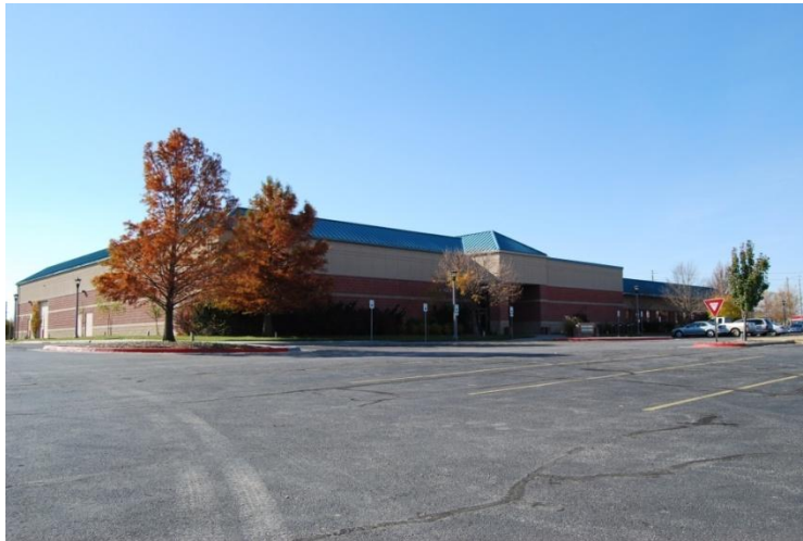
4H Extension Offices
